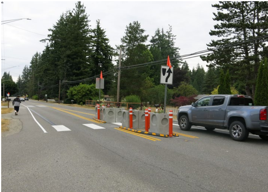
Quick Build Pedestrian Crossing, Seattle
