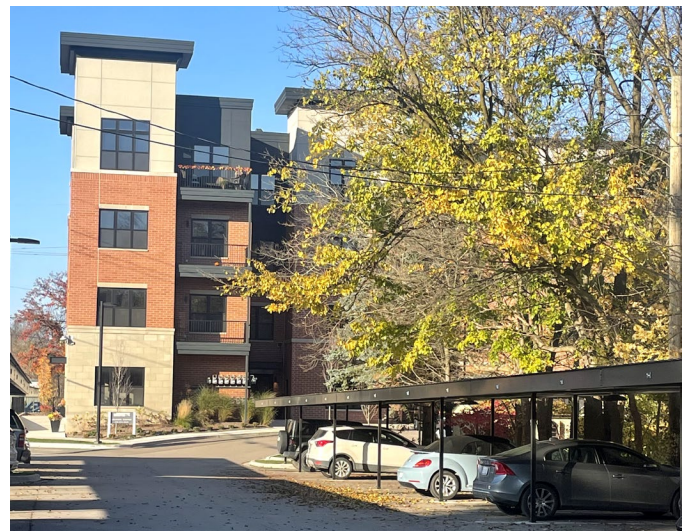
The Marquette apartment building on Washington Street
